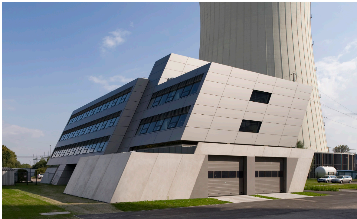
E.ON power plant in Zolling Administrative building in an "inclined position"
